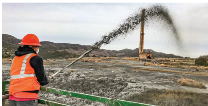
The grey areas are the aluminum dross—contaminated soils that we covered. Dross is a byproduct of the aluminum smelting process.
