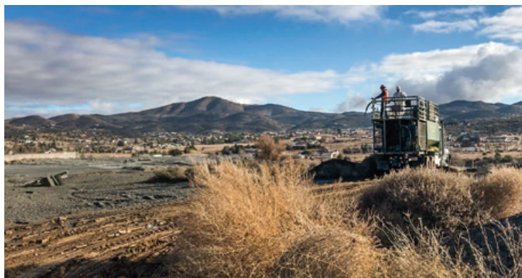
The grey areas are the aluminum dross—contaminated soils that we covered. Dross is a byproduct of the aluminum smelting process.
